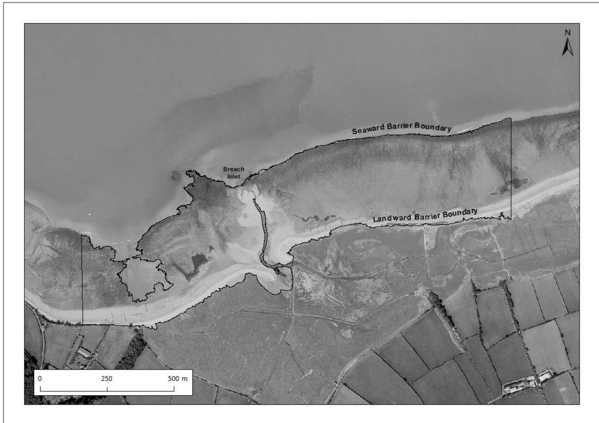
Figure 2. Aerial photo showing and labelling the breach, landward boundary and seaward boundary (Image from Channel Coast Observatory, 2010).
