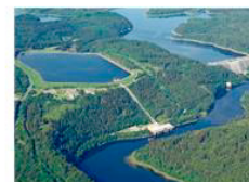
Figure 2) Vattenfall's Wendefurth PHS site. Image source: Renewis.biz
