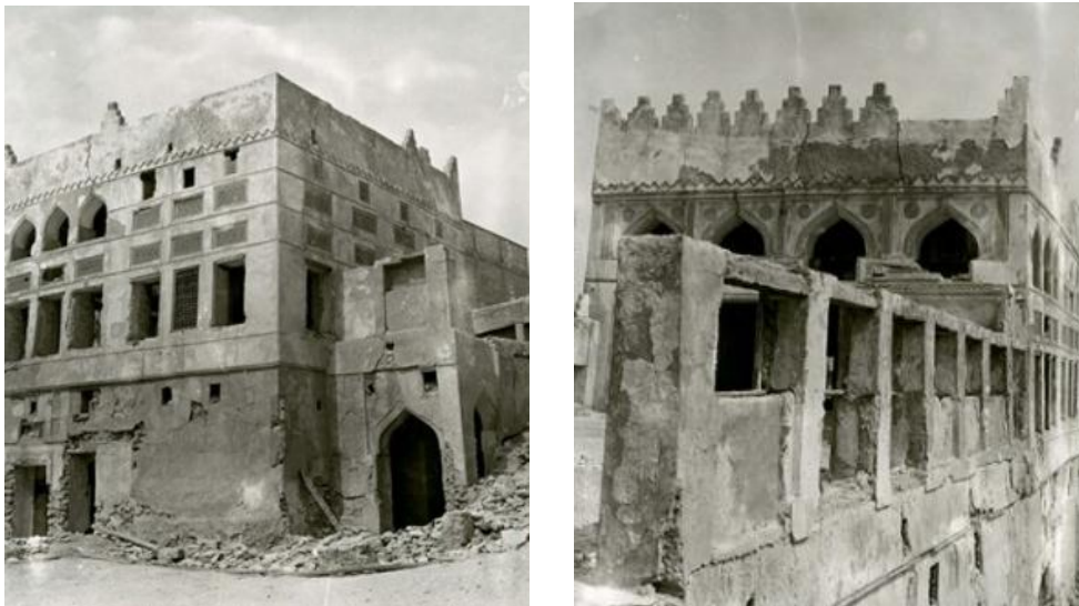
Fig 5.5 Photographs of the Sheikh Hamad house in ruins, prior to its demolition.
