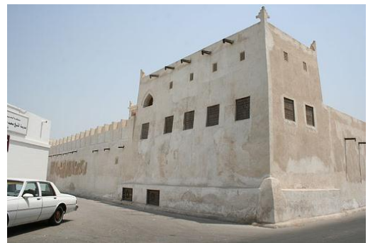
Fig 2.8.d Sheikh Isa bin Ali House
