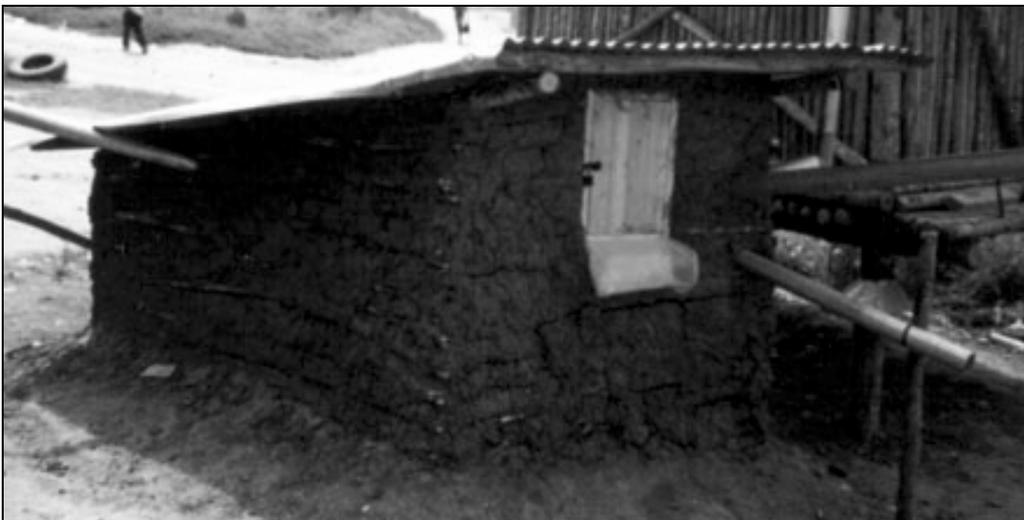
Lowering construction quality from a high standard initially mainly affects appearance. The next parameter to suffer is durability – cheap materials like wattle and daub walls do not have the durability of mortar and will need more frequent renewal. Finally the point is reached where water quality itself is degraded, for example by omitting the cistern' s cover.
