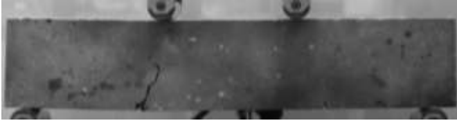
Fig. 1. A failed concrete beam sample
