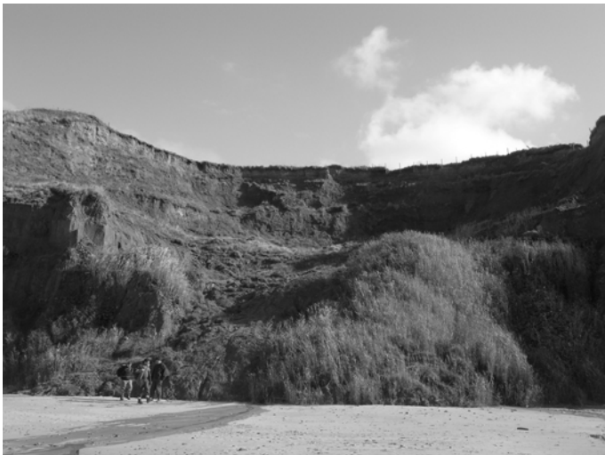
Figure 6. Kettle hole failure in silts at [230650 340955].
