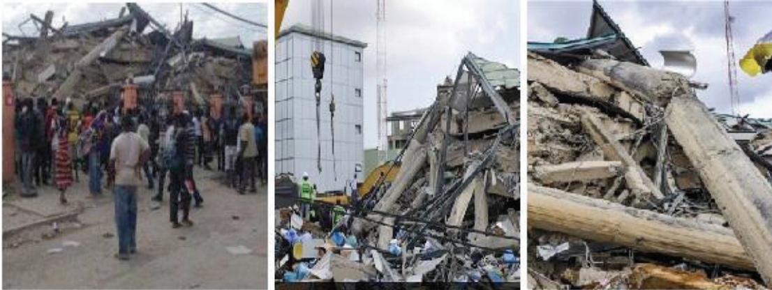
External View of Building after Collapse
