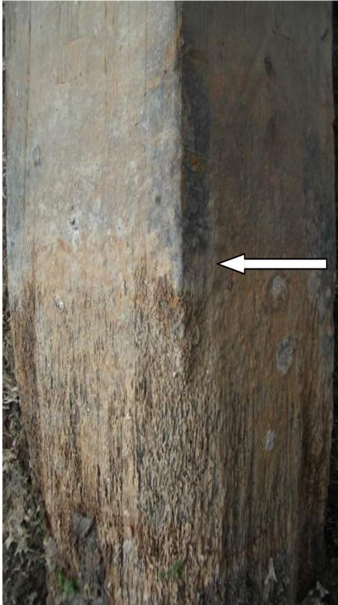
Figure 2: Waisting of timber pile, i.e. it develops a waist (or a pencil point shape) in the intertidal zone, caused by limnoriid attack. Note that there is no attack below the sea bed line which is indicated by the arrow.
